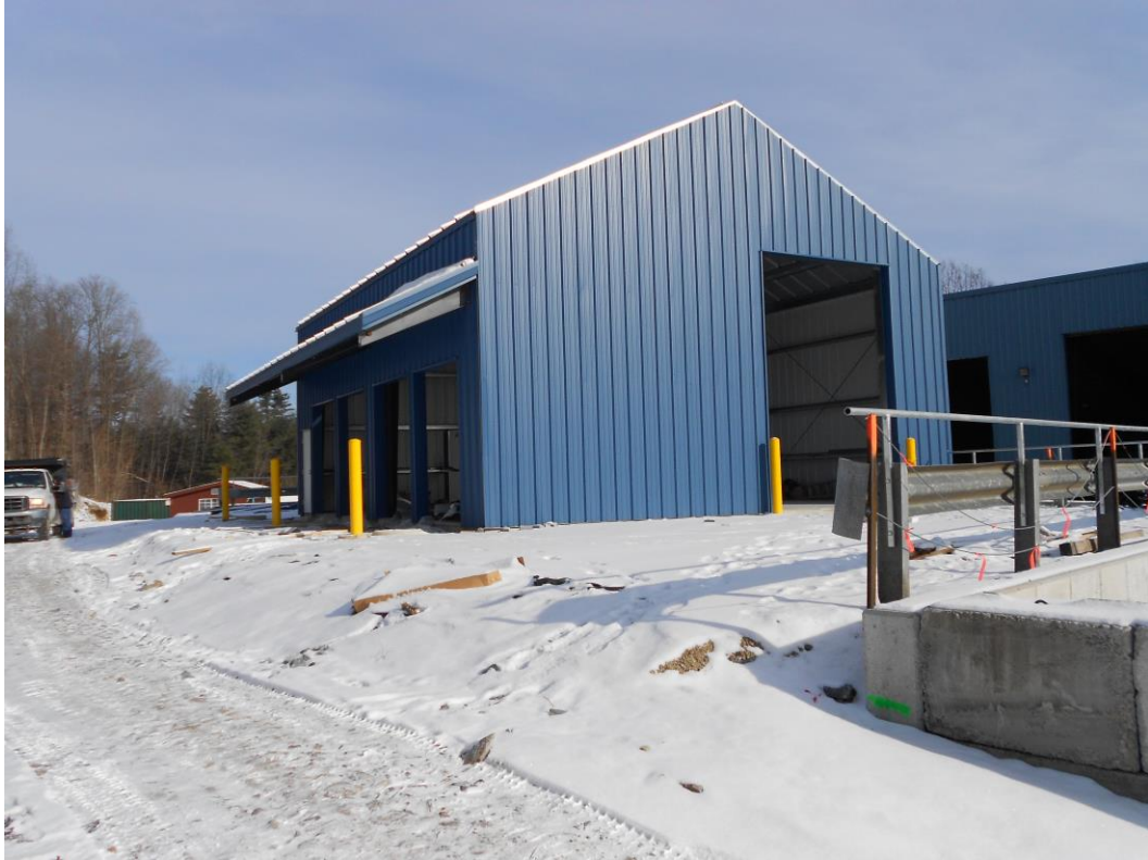
ACSWMD Transfer Station, Middlebury, VT - New Special Waste Building Construction 2014
